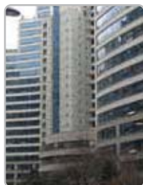
LG Display Building in Gumi City
